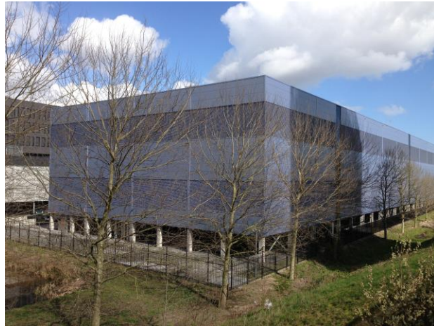
The location of our new Amsterdam datacenter.
